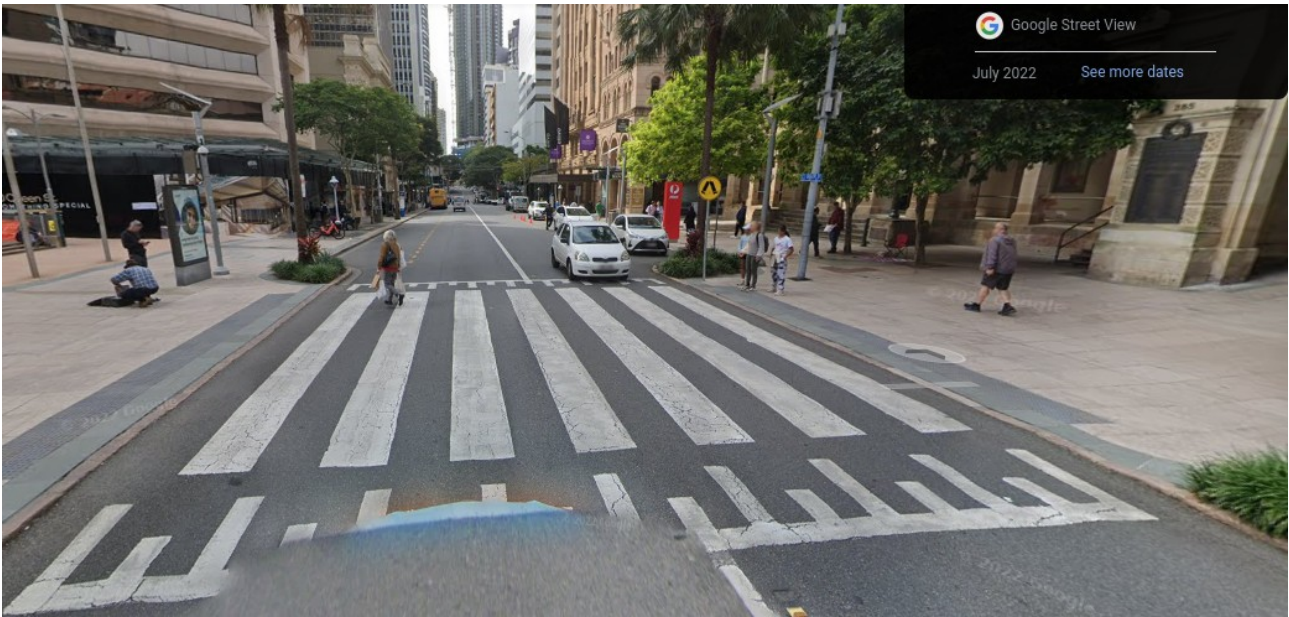
Figure 3: Post Office Square pedestrian crossing, circa July 2022. Photo from Google Maps. The “wombat” crossing is flush with the pavement and raised up from the level of the road.
